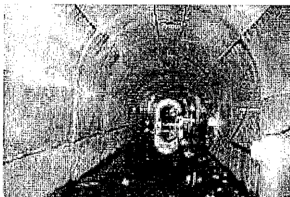
PIC ( Polymer Impregnated Concrete ) 版
